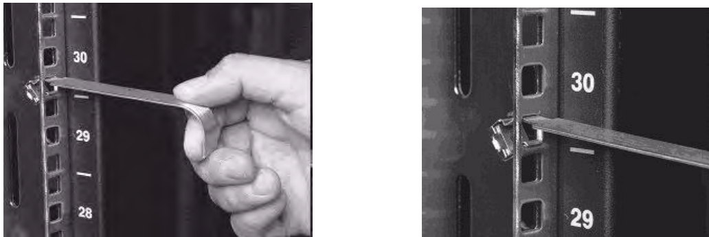
Figure 3-22: Installing the Cage Nuts
