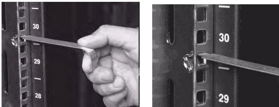
Figure C-32: Installing the Cage Nuts
